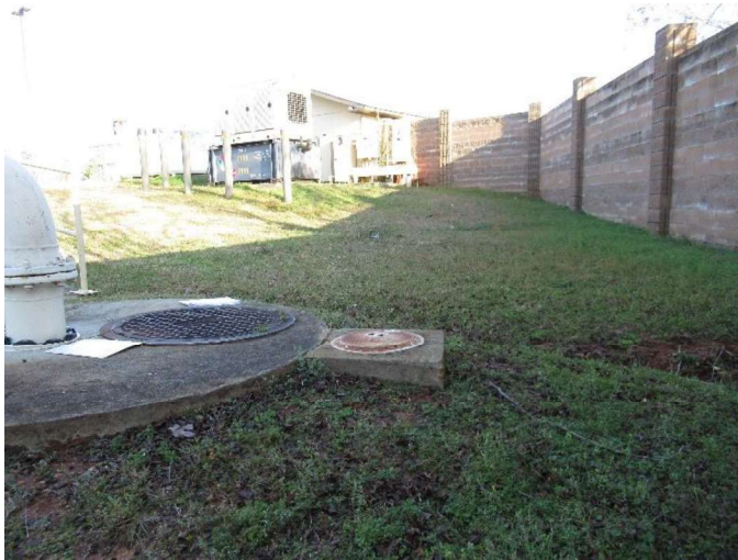
Housekeeping Pad on Plan North Side of Shaw Drive
