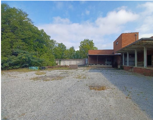
Photo 1: View of the southwestern side of the Site building.
