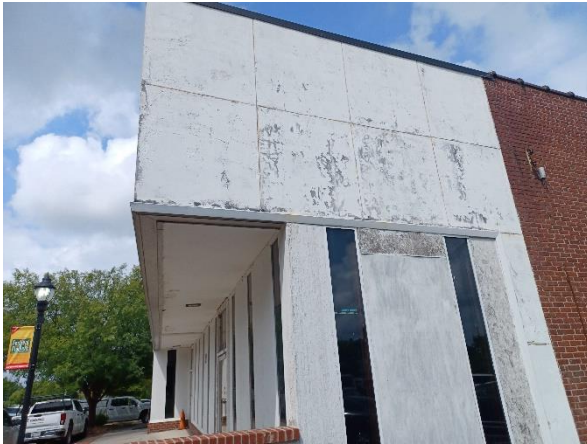
Photo 19: View of the white plaster skim coat and gray plaster base coat on the southeastern exterior of the building.
