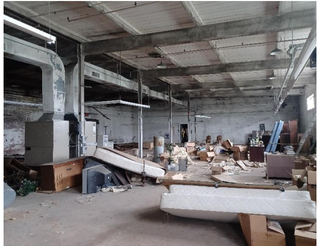
Photo 8: Typical view of the warehouse.
