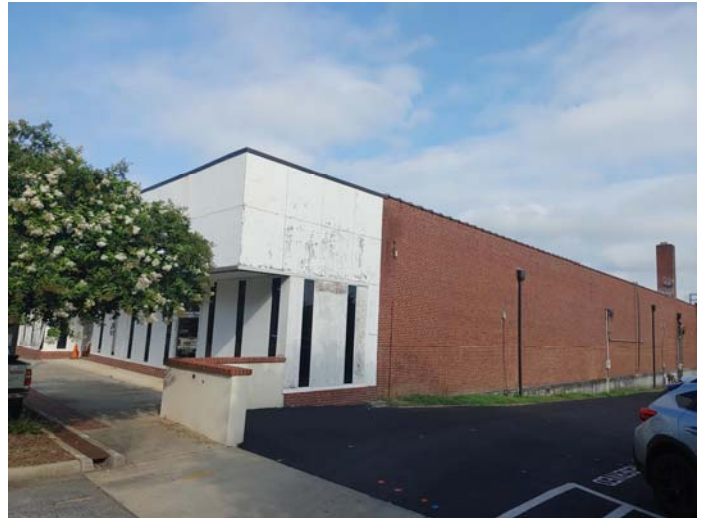
Photo 4 – Typical view of the right side of the building (side D)
