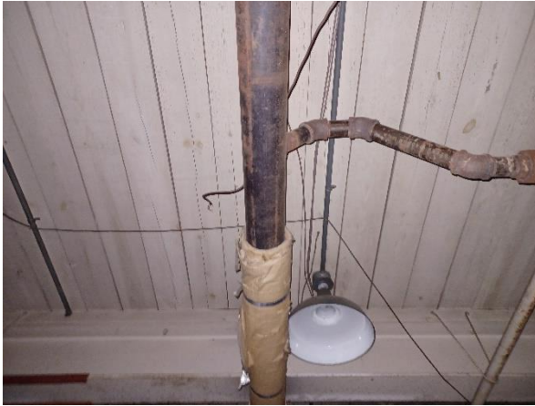
Photo 21: View of the tan tarpaper with underlying black mastic in the basement.
