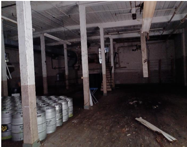
Photo 9: Typical view of the warehouse.
