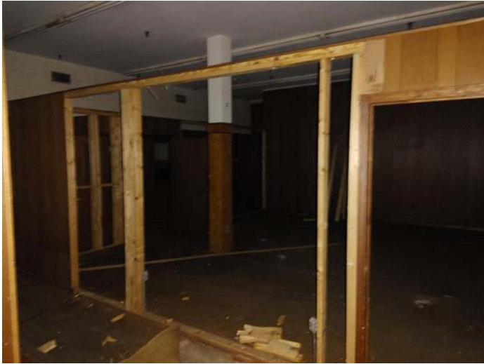
Photo 13 – Typical view of the office area
