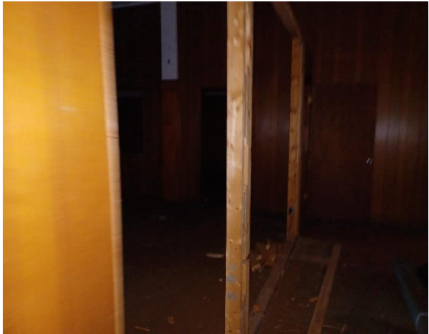
Photo 7: Typical view of the office area.
