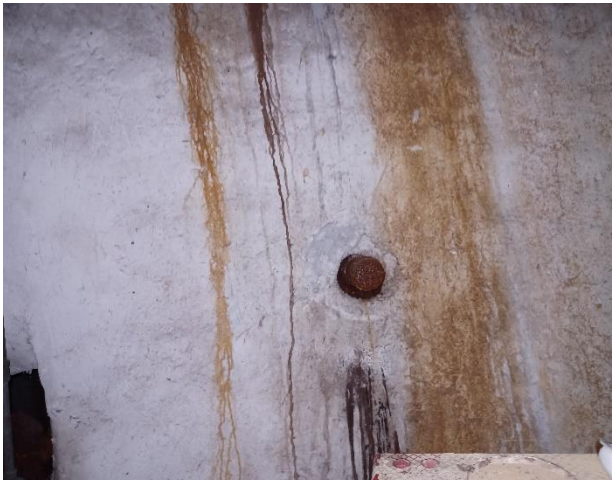
Photo 23: View of the asbestos containing gray insulation on the furnace in the basement.
