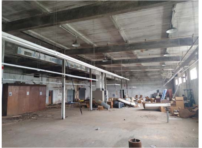
Photo 14 – Typical view of the back warehouse area
