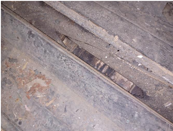
Photo 17: View of the black tarpaper underneath the hardwood floors in the showroom, office area, and warehouse.
