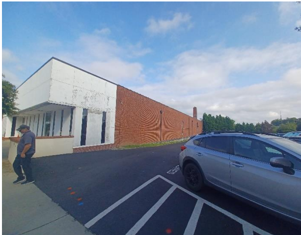
Photo 3: View of the eastern side of the Site building.
