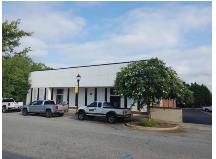
Photo 2 – Typical view of the front of the building (side A)
