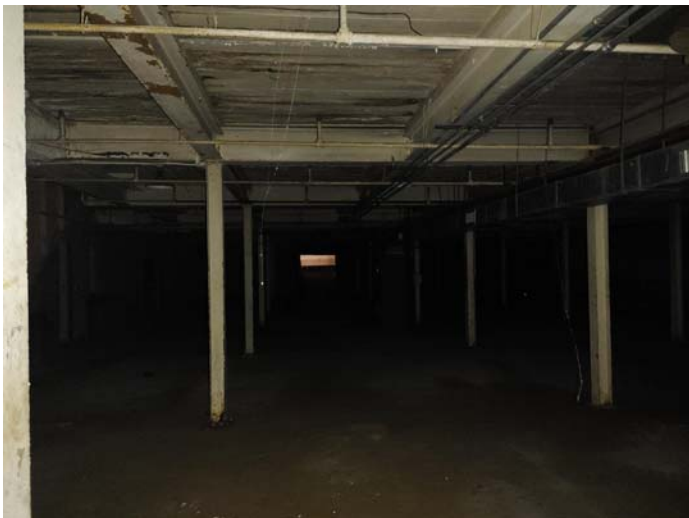
Photo 15 – Typical view of the basement with no LBP ceilings
