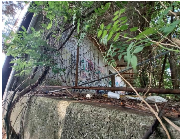
Photo 4: View of the northern side (back) of the Site building.
