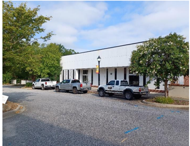
Photo 2: View of the southeastern (front) side of the Site building.
