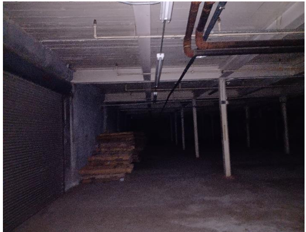
Photo 10: Typical view of the basement.
