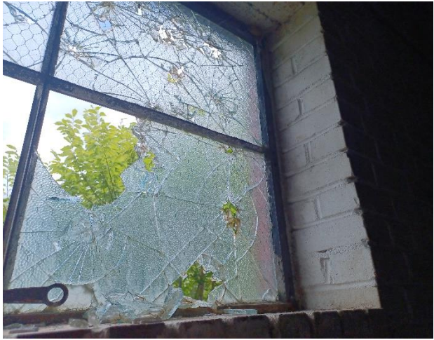
Photo 25: View of the white glazing on the warehouse windows.
