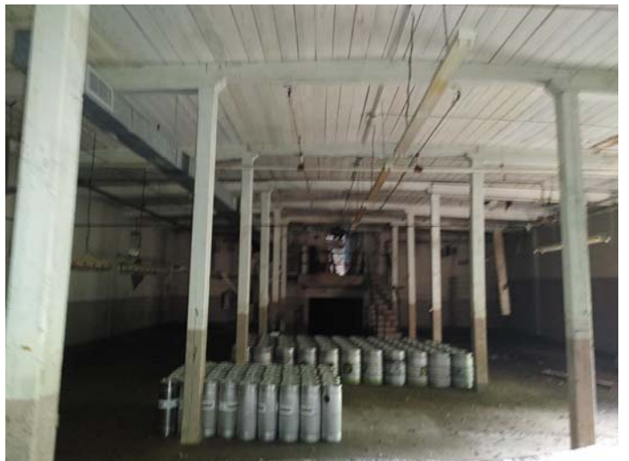
Photo 16 – Typical view of the basement with LBP ceilings
